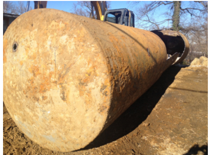
One of the water holding tanks from the pump house.
